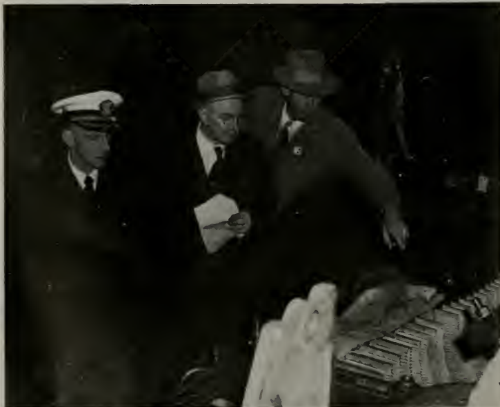
Bethlehem's Yard Manager T. C. Ingersoll explaining turbine reblading job to Pacific Marine Review Editor, T. D. McMullen and Navy Captain Donald L. Irwin, Supervisor of Shipbuilding at Bethlehem.
